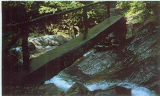
This rustic bridge is constructed of only natural undimensioned materials appropriate for Semi-Primitive settings.
