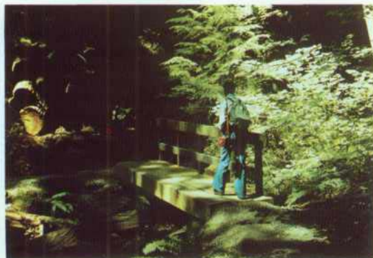
This simple rustic bridge is made of natural, but dimensioned, materials appropriate for a Roaded Natural setting.
